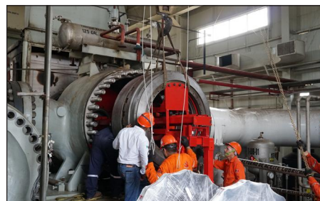
Figure 3: Flexware service personnel reassembling a Rolls Royce RF2BB-36 Compressor in Cempoala, Mexico following a reate to improve gas delivery service. Credit: Flexware Inc.
